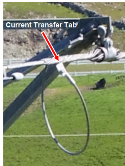
PLP Suspension (this does not have a grounding lug position; it utilizes what is called a "current transfer tab")
