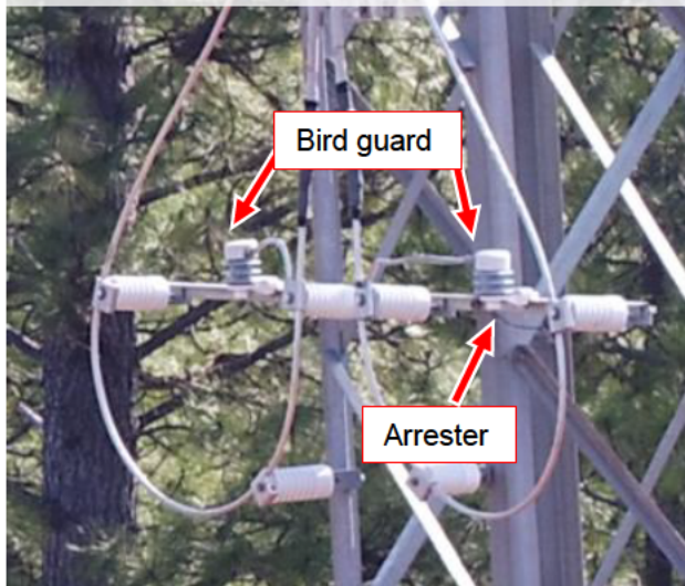
Correct Installation of Lightning Arrester
