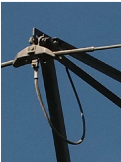
AFL Suspension (ground lug located at the bottom of suspension)
