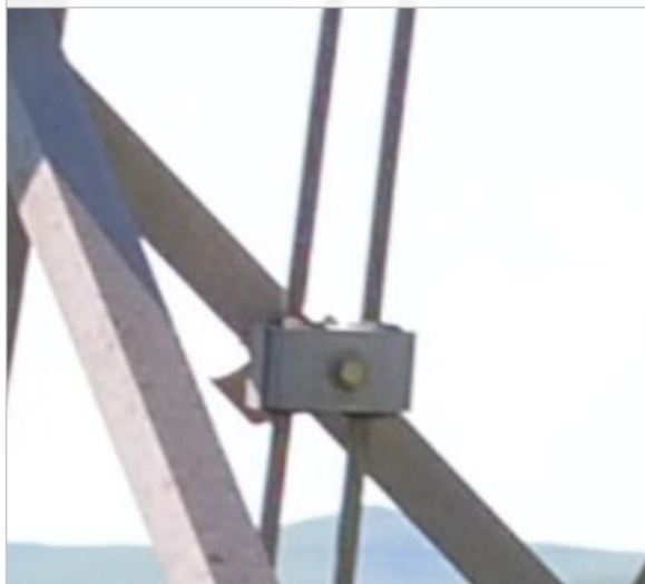
Correct Installation of Down-Lead Clamp
