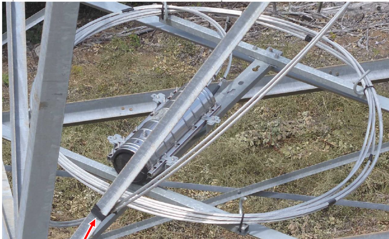
Tape attaching OPGW to tower member
