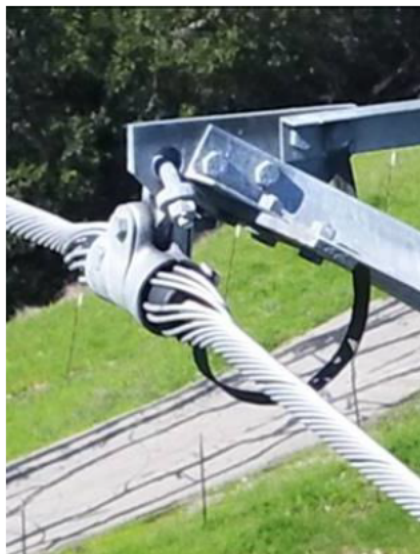
Dulmison (ground lug on the back side of suspension)
